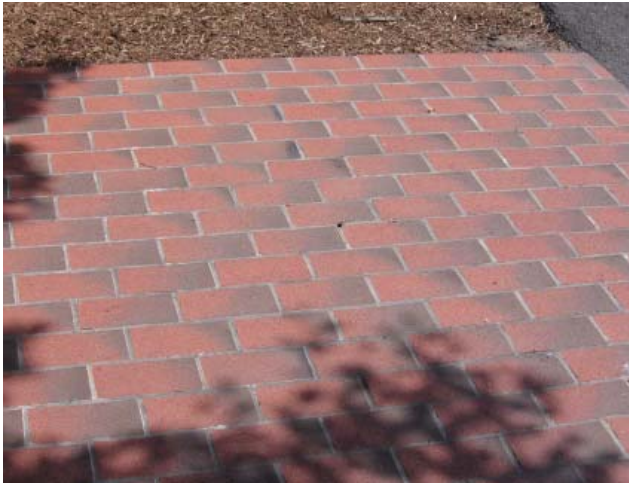
Photo 1 Clay Pavers in a Mortar Setting Bed
